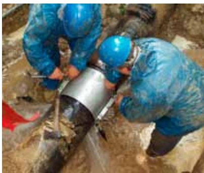
Repair clamps being installed. Sent in by Petr Kvicerá, AVK VOD-KA.
