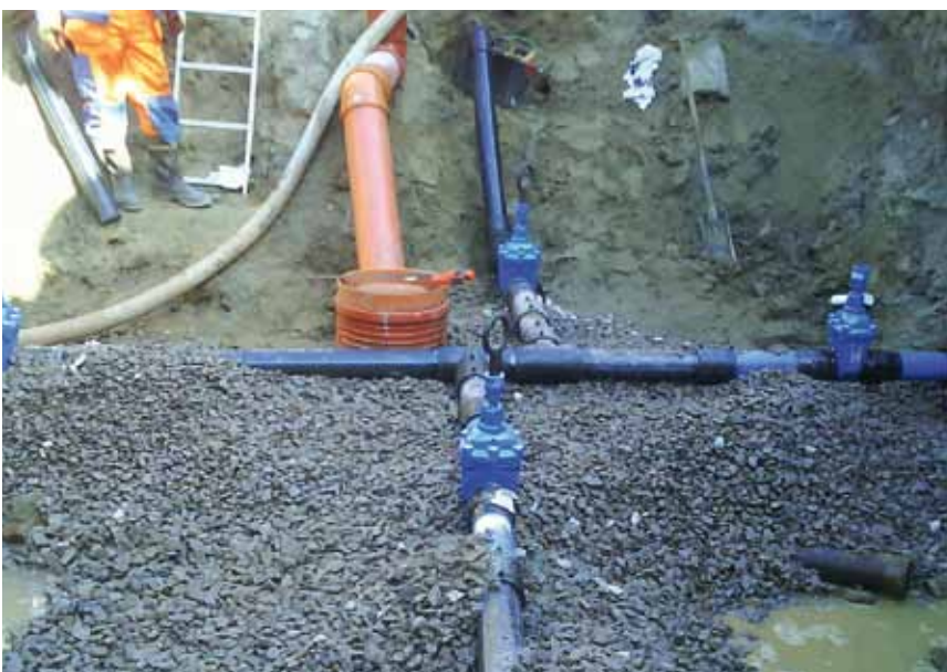
Gate valves in Kalix. Sent in by Åke T in Kalix, Sweden.
