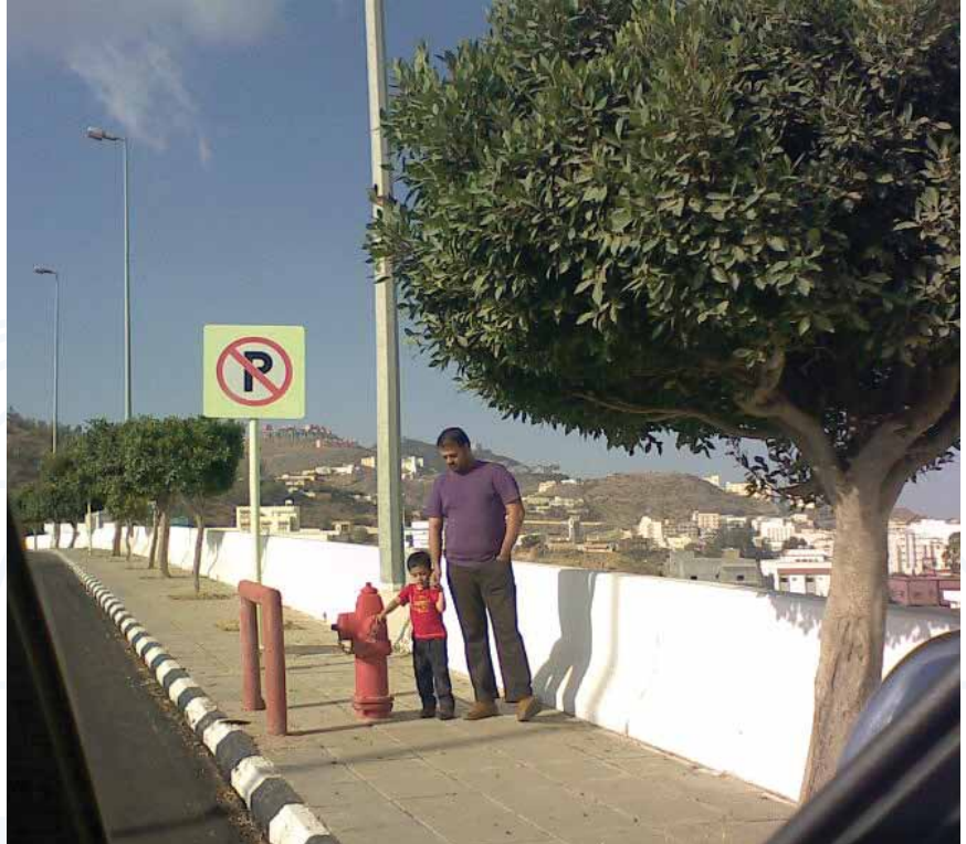
Series 27/00 dry barrel fire hydrant on a hill Station in Saudi Arabia, called Al-Baha-It is at an height of 2500 meters above sea level. In the picture Imran Shaikh, Quality & IT Mgr., AVK Saudi Valve Mfg. Co. Ltd., Jeddah, Saudi Arabia and his son Omair.
