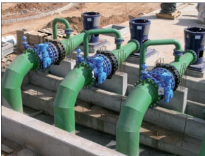
Double eccentric butterfly valves in Portugal. Sent in by Vanessa Martínez, AVK Válvulas SA.
