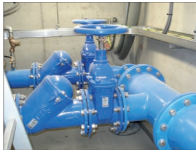
Gate and ball check valves in Holland. Sent in by Hans Bos, AVK Nederland BV.
