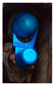
Existing hydrant with AVK device fully installed. Note the outlet and operating cap now fully protected
