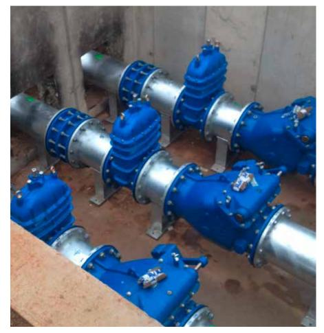
A pit construction at Frogmore site where the AVK valves have been installed
