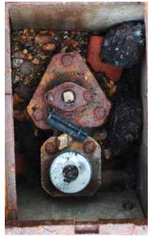
Existing hydrant with outlet security device installed
