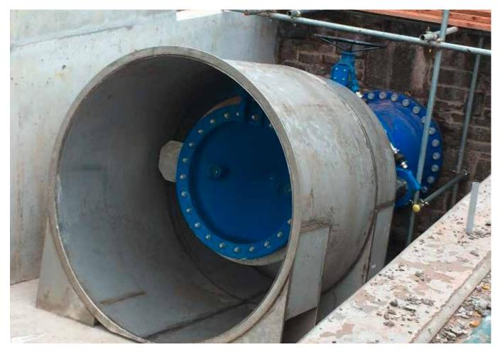
Picture 1: Free discharge valve and hood installation
