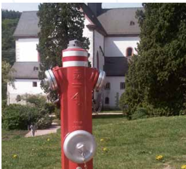
Installation of af series 84 fire hydrant in Rheingau, Germany.
