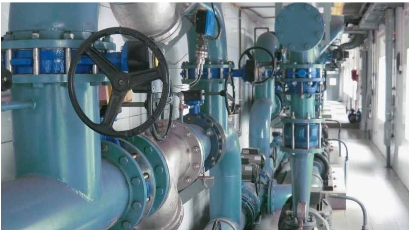
AVK butterfly valves used at Suez in Macao, Da Shuitang Water Plant.
