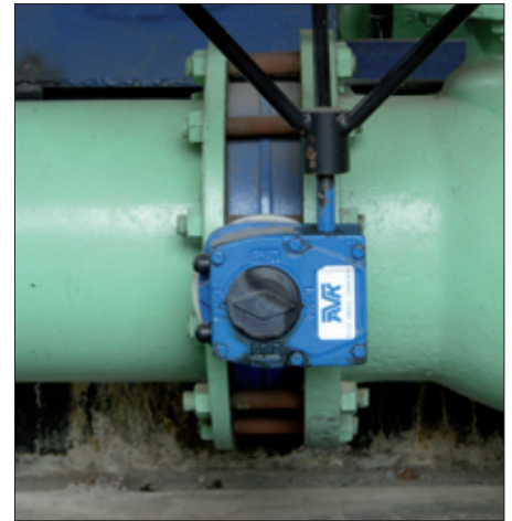
AVK butterfly valve c/w gearbox, series 75/10 (Wafer Type).
