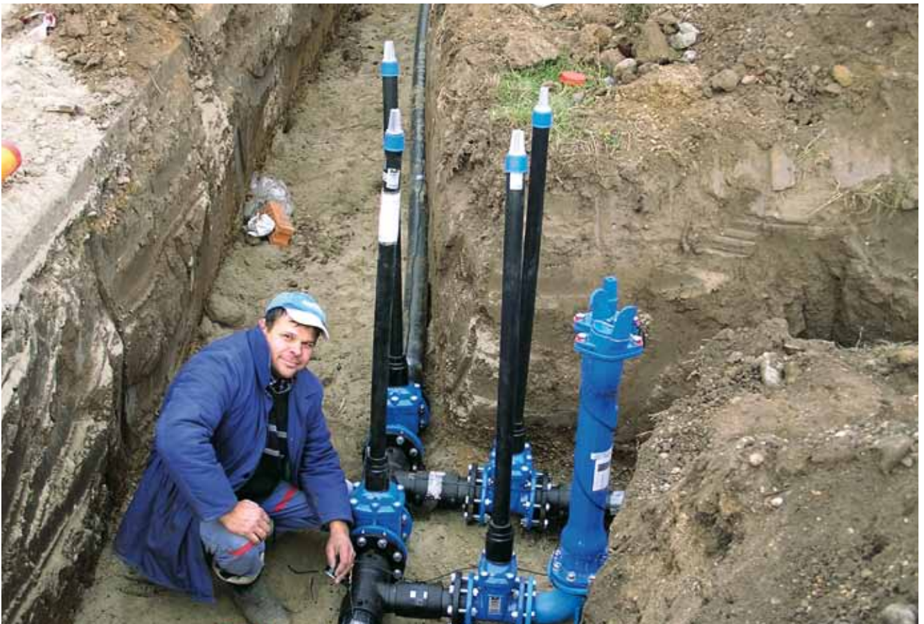
Project in Slovakia, series 06/30 gate valves, series 04 extension spindels and series 35 hydrant - sent in by Libor Tóth, Slovakia
