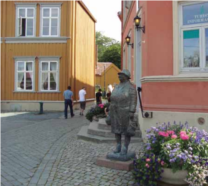
An AVK Victoria hydrant in a square in Trondheim Kommune, Norway - sent in by Sverre Tage Austmo, AVK Norge AS
